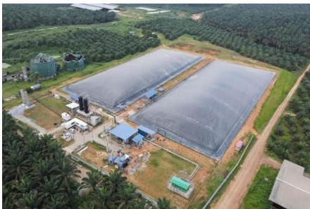
MTC Orec's biomethane generation plant in Sedenak, Johor.
