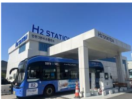
A hydrogen charging station [INCHEON GOVERNMENT]
